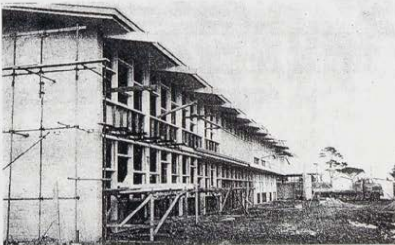
Recent view of the New Preparatory School
