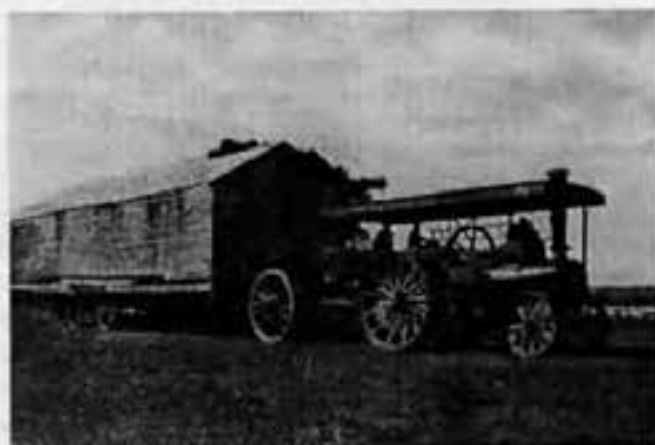
11. One bay of the shed hauled by a steam traction engine from Marnockvale to the present site.
