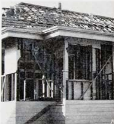
First stages of demolition
