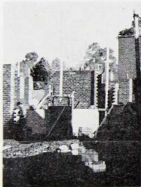
Early stage in erection of new library/resource centre
