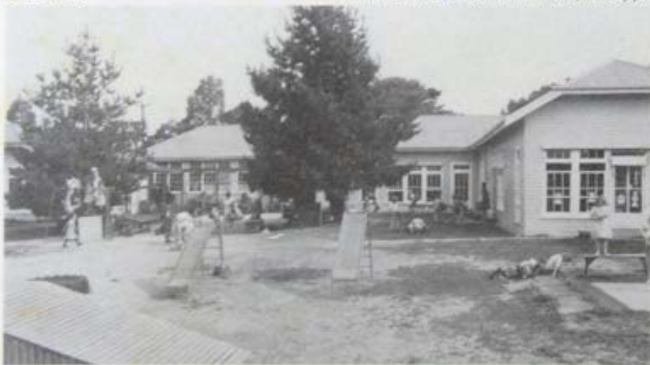
The original kindergarten class-room (centre) has now been extended with class-rooms on each side. The photo depicts only a portion of the total Campbell House complex.
