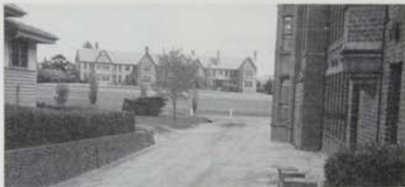
Mackie House from near the Hospital before the Coles Wing was built.
