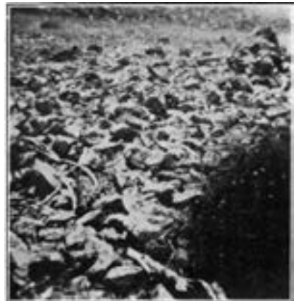
ONE OF THE HEAPS OF STONE CHIPS. TYPICAL OF MANY.
