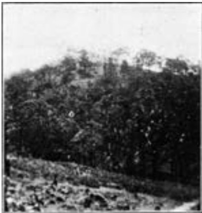
SITE OF THE QUARRIES,
